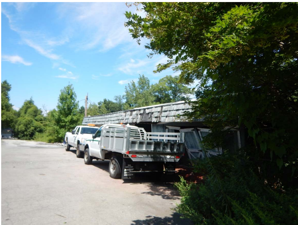
Photo 16. View looking north within the Nilson Greenhouse complex. The main building is visible to the right in the photo.
